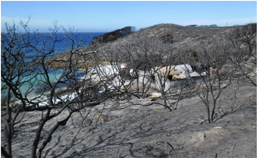
17. Drages Beach, December 2012. Shack destroyed by fire.
