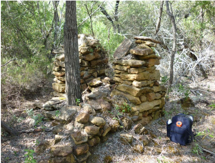
4. Old chimney 2015, from shack built c1873. It is c500m SW of Peppermint Dam.
